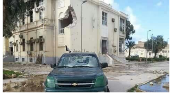
BDD in 2014 partially damaged
